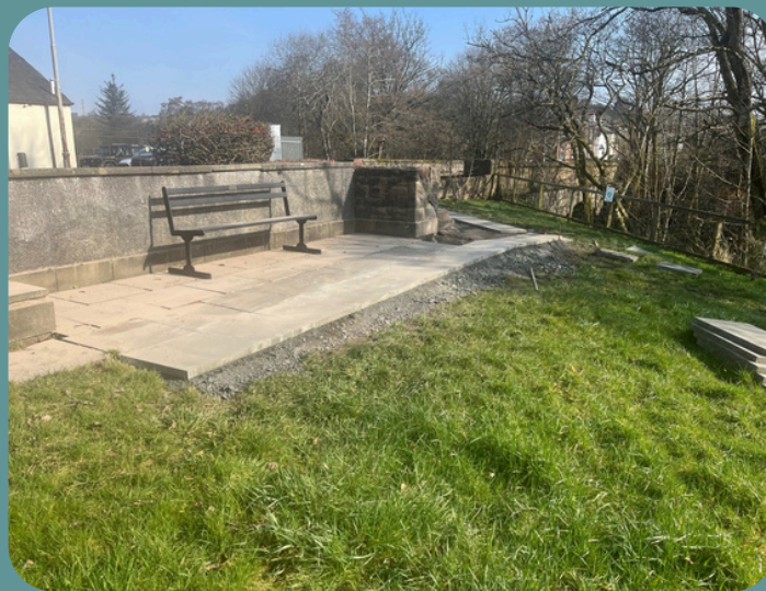
Here is the refurbished paved area and new access to the bench at the East Main Street end of the Waterlip. Funding provided by Walking Scotland
